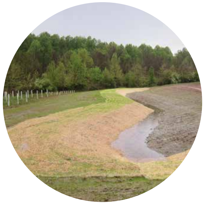
A newly constructed level-lip spreader captures runoff from the adjacent farm field. Photo: Stephanie Eisenbise
