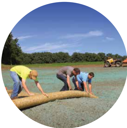
Erosion control matting is unrolled to stabilize the land on which a level-lip spreader was installed in summer 2016. Photo: Kay Dixon
